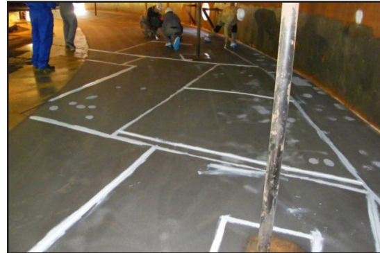
Application of the stripe coat to all weld seams
